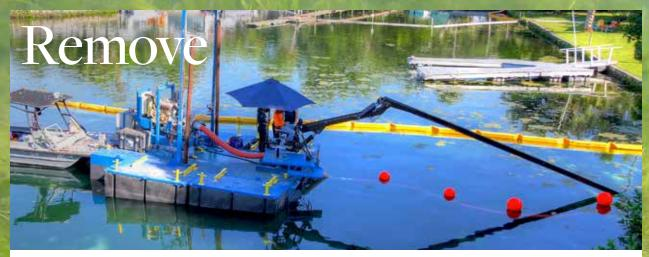
*Lyngbya* is hydraulically vacuumed from the river bottom and transported to land via floating hoses for processing.
